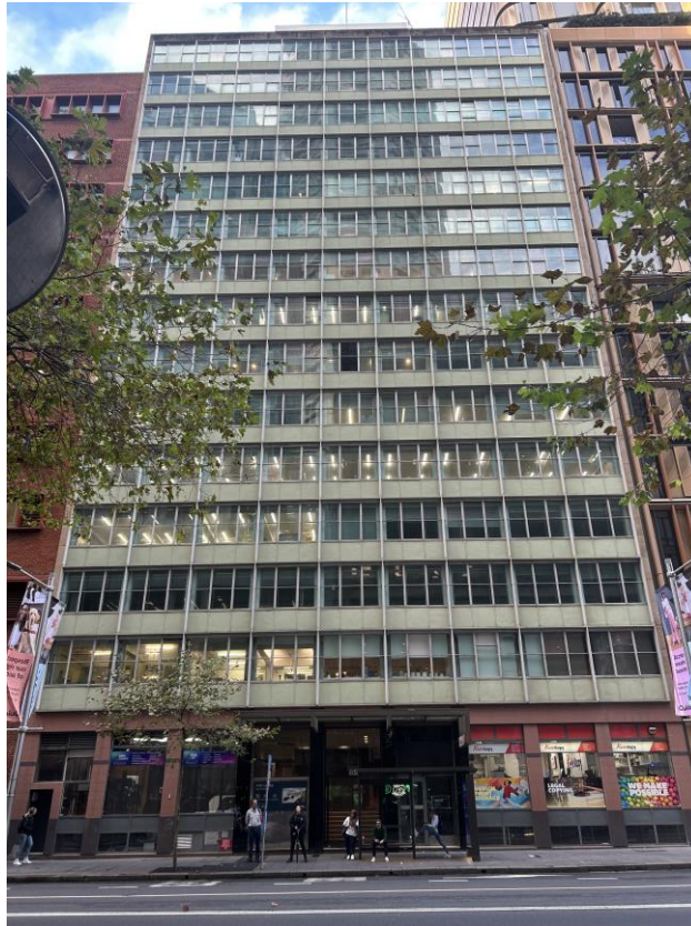
Figure 1: 82-88 Elizabeth Street, Sydney, viewed from the east
